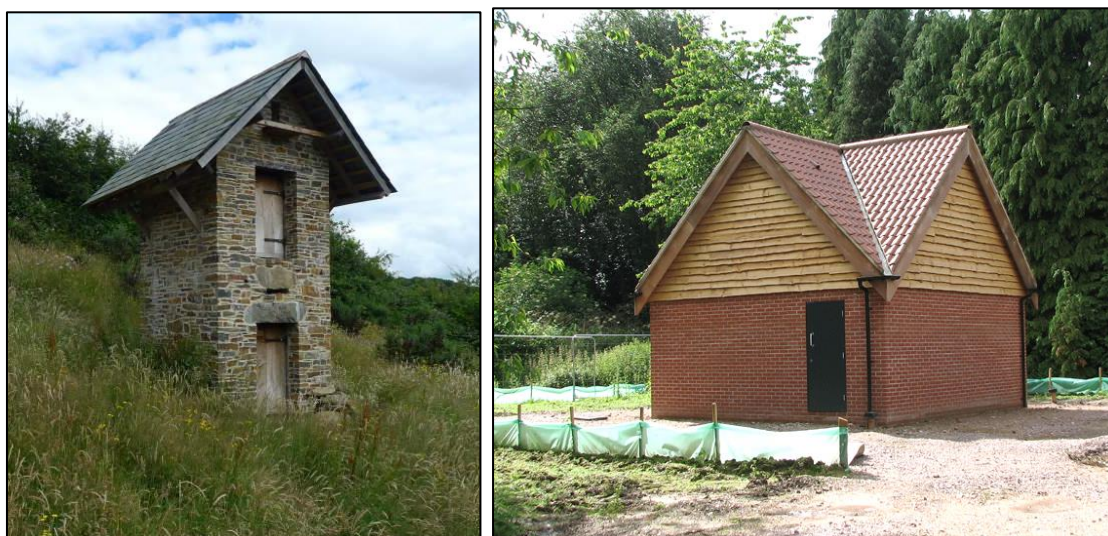
Figure 9. Example of a wildlife tower and waney-edge cladding modifications for bats.
